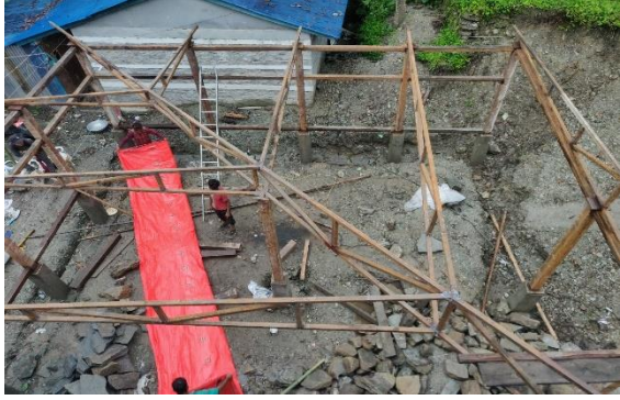
Steel Truss work at the dining area
