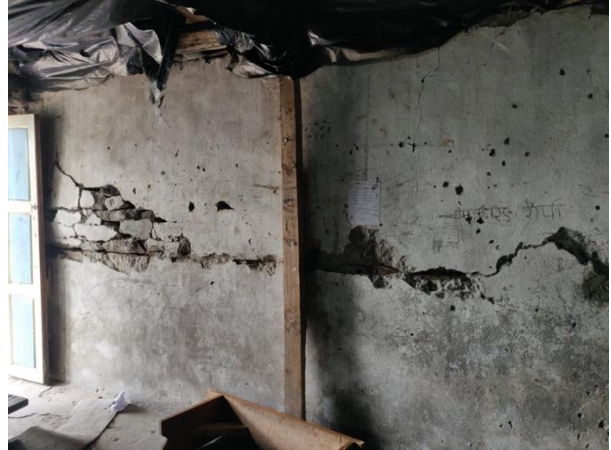
Cracks made by the earthquake on the ground floor
