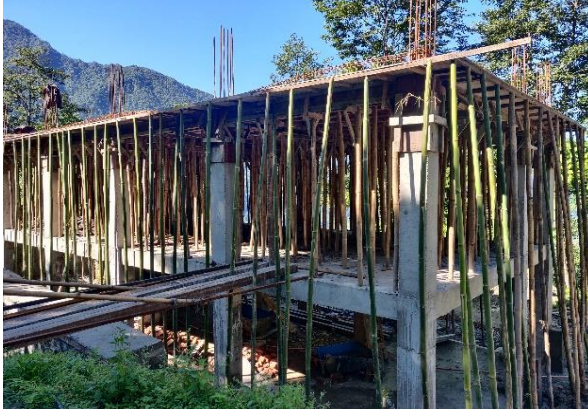
Suturing preparation for top-floor Slab
