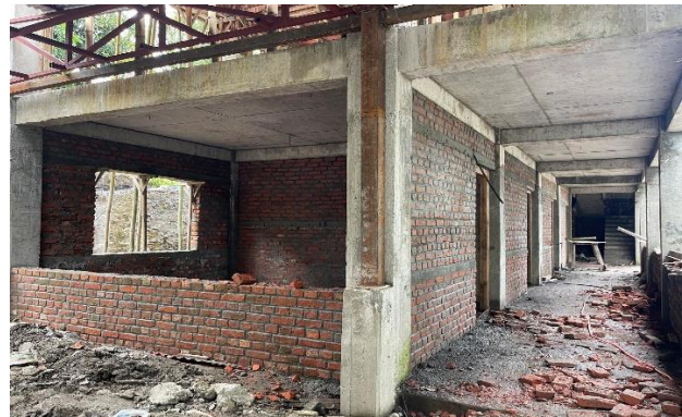
Brick masonry wall work on the ground floor
