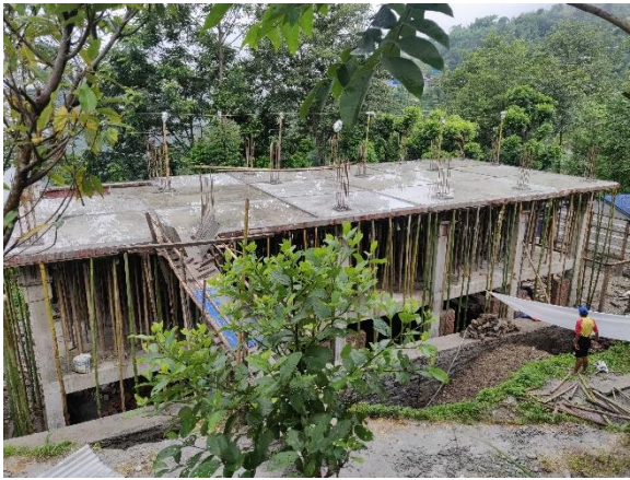
Slab cast of top-floor
