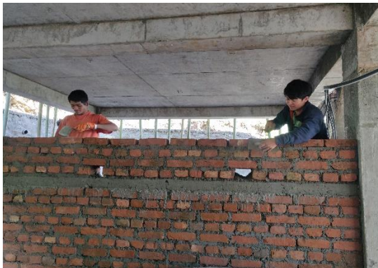
Brick masonry wall work on the ground floor
