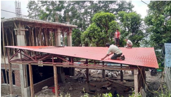
CGI roof installation of the dining area
