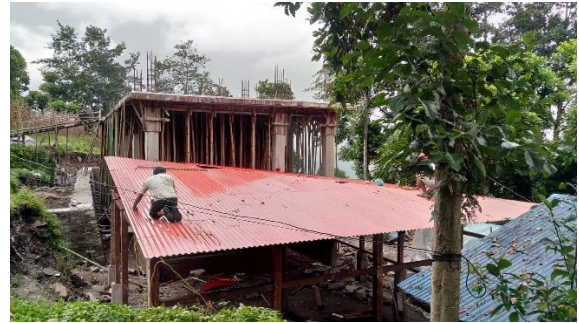
CGI roof installation of the dining area
