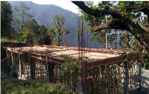
Suturing preparation for first-floor Slab
