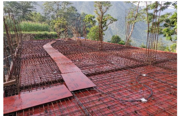
Reinforcement setting for first floor Slab
