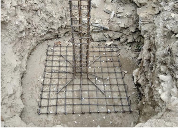
The setting of Reinforcement in the column at the foundation
