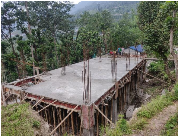
Completion of first-floor slab
