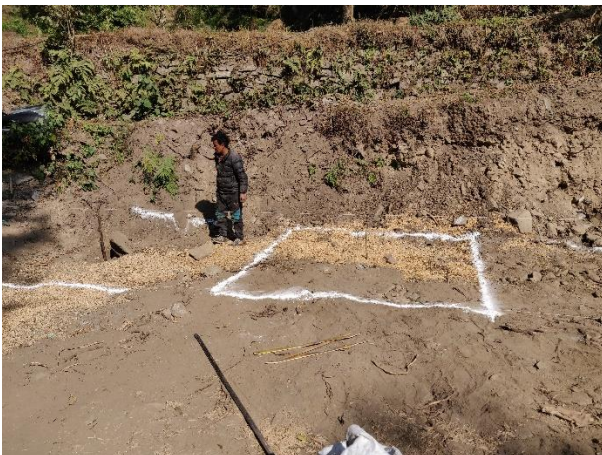
Tranch Setting for the foundation work
