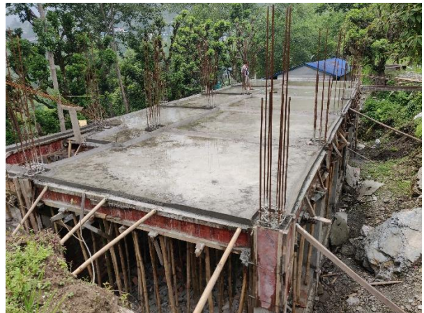
Curing of the slab after completion
