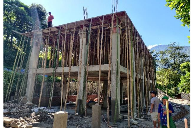
Suturing preparation for top-floor Slab
